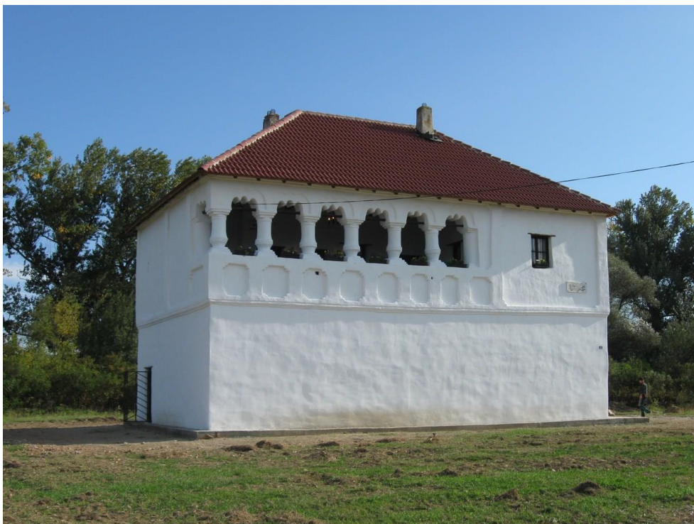
Fig. 3. The condition of the cula in 2010.
